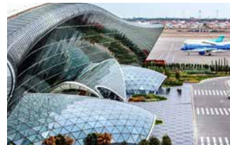
Baku International Airport Azerbaijan
