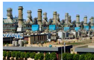
Suleymaniya Combined Cycle Power Plant - Iraq
